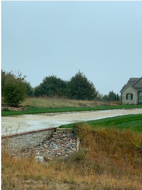
View of driveway headwall
